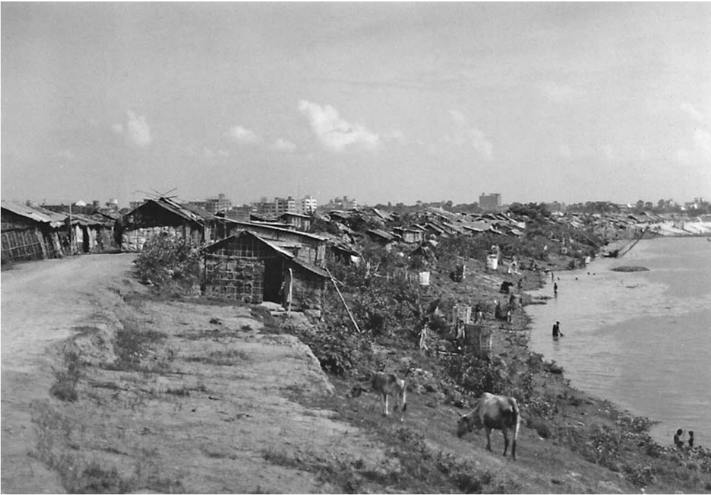
Photo 3.17: Multipurpose embankment with erosion. Source: Alan Bird
