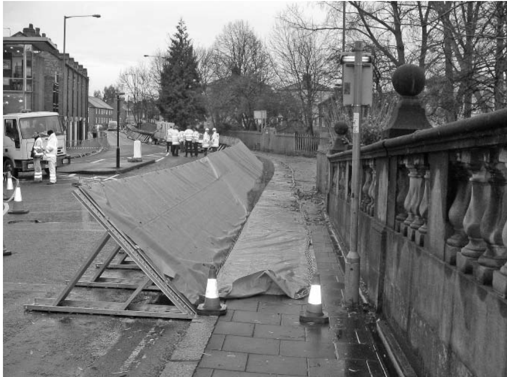
Photo 3.15: temporary flood barrier deployed. Source: J Lamond
