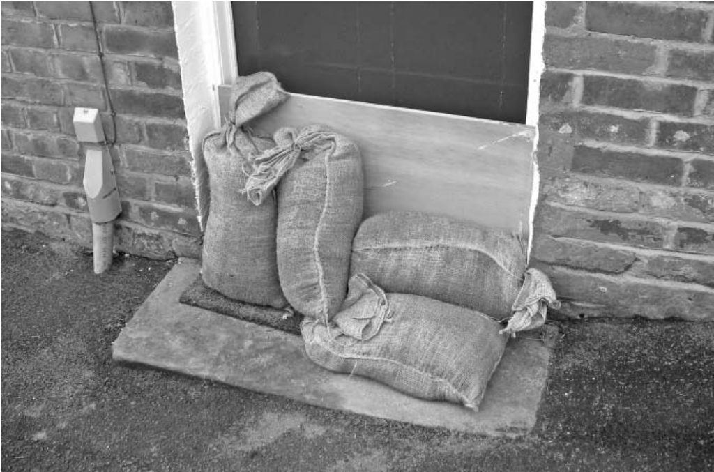
Photo 3.16: Homemade door guard. Source: J Lamond
