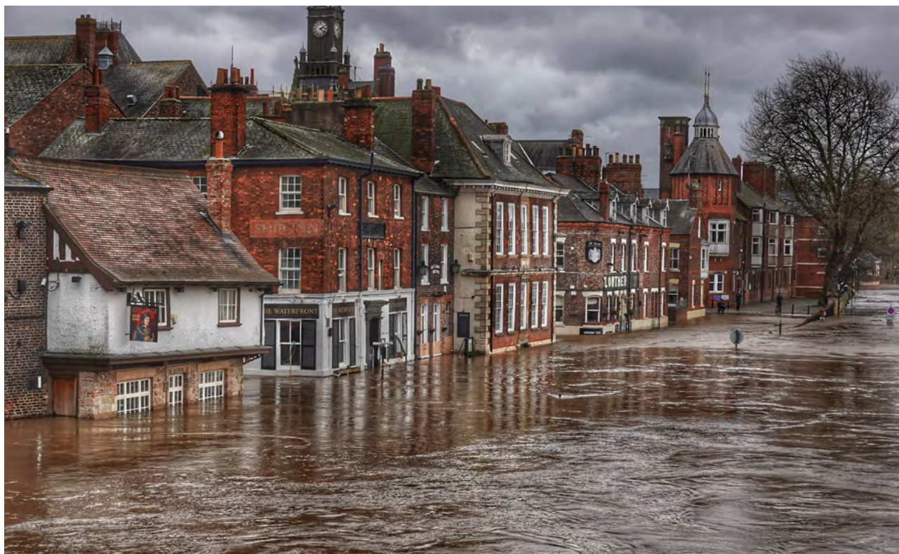
Flooding caused by Storm Dennis, 2017
